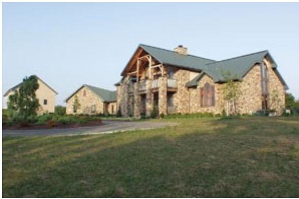
Photos courtesy of Donald B. Smith Roofing Inc., Hanover, Pa.
