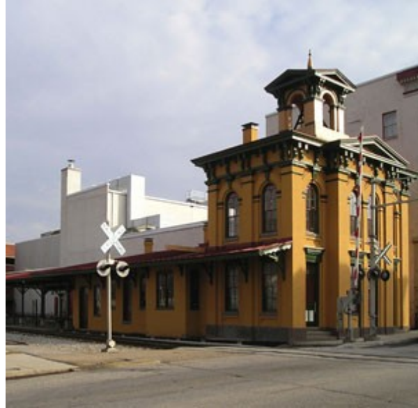
Donald B. Smith Roofing Inc., Hanover, Pa., installed a new roof on a historical railroad station
